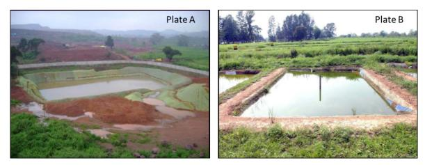
Plate 8.10 (A and B): The Geogreen blanket used for protecting the slopes and base of the storage tanks dug on the ground to store rainwater (Courtesy: Sri Venkateshwara Fibre Udyog, Bangalore)
